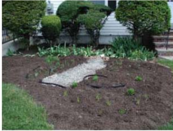
At time of installation
